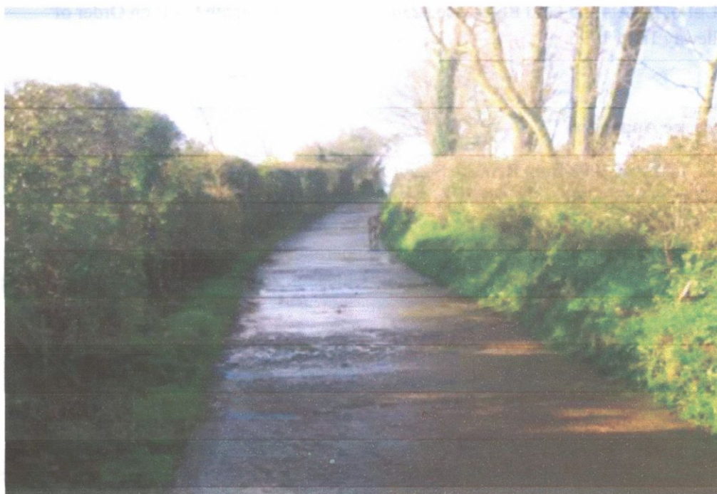
Section of Bridleway under dispute – concrete laid in 1943 still in place in 2015
